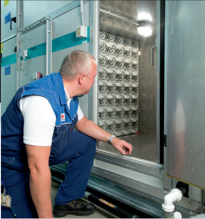
View into the humidification section equipped
