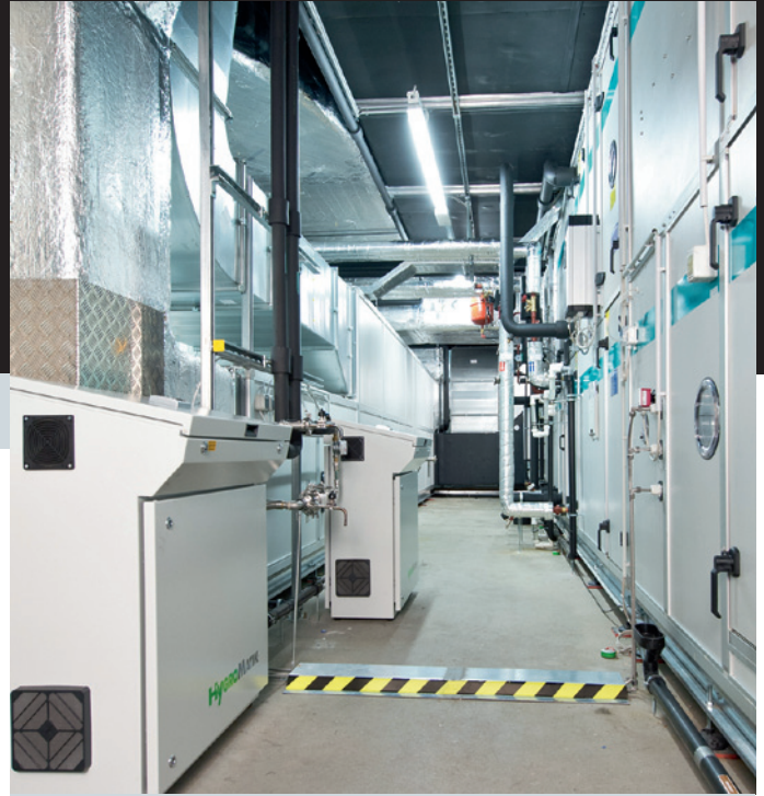
Technique room in the Blutzentrale (blood centre) Linz with two HygroMatik HDS systems
